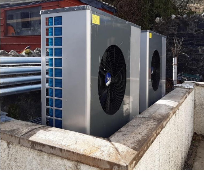
Images of ASHP at Arrochar PS and Strachur PS
